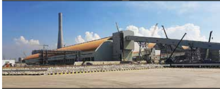
Matarbari Coal Power Project
